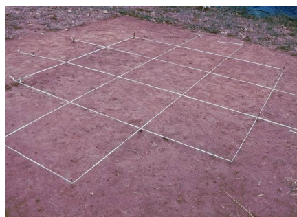
图4 现场定位、放线 Fig.4 Fixing and mark position
