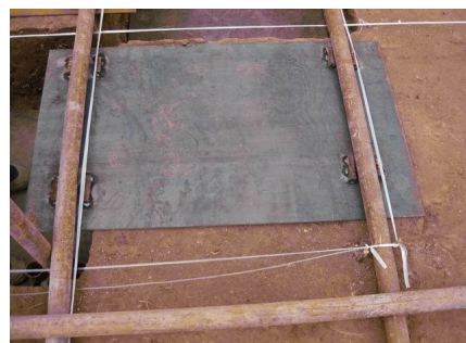
图6 安放托换顶板 Fig.6 Installing top slabs underpinning slabs
